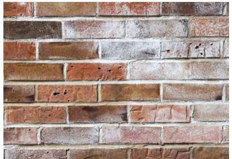
Efflorescence seen in the brick
