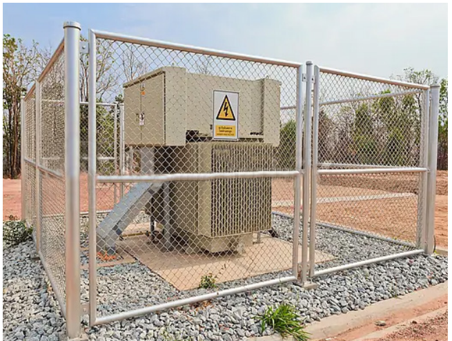
Fenced power transformer
